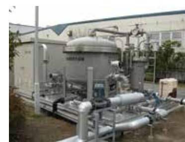
800m 3 / day Industrial-to-drinking water installation (Meat processing plant)
