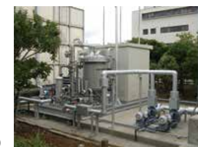
800m 3 / day Industrial-to-drinking water installation (Meat processing plant)
