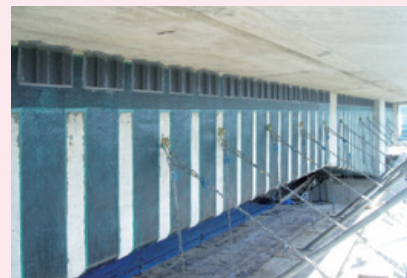
Genta Bridge under construction
