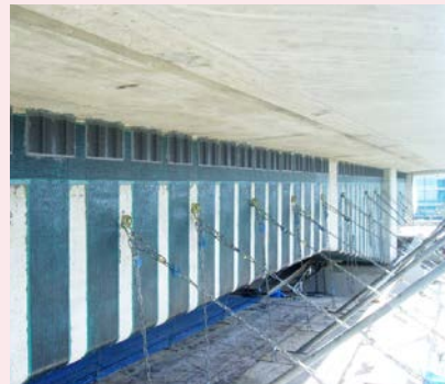
Genta Bridge under construction
