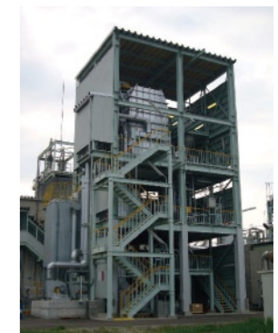
Chemical recycling plant
