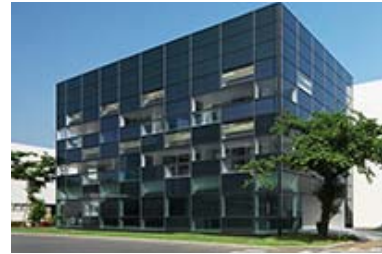
External view of the ZEB Verification Building
