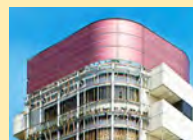
Example of an application for amorphous silicon thin-film PV modules JR Meguro Green Building (Shinagawa-ku, Tokyo) Client: JR East Building Co., Ltd.
