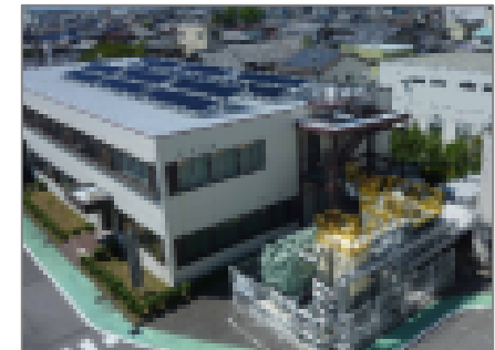
Verification facilities at Naoetsu Plant
