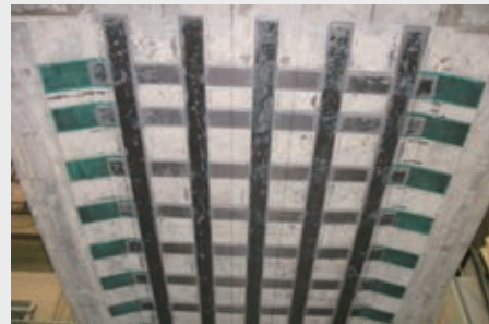
Deck slab reinforced with e-Plate
