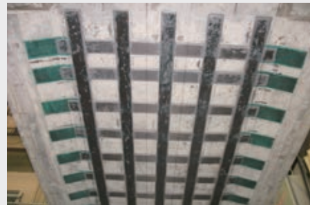
Deck slab reinforced with e-Plate
