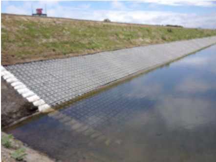
The Kawauchisawa River where GOBIMAT™ was laid.
