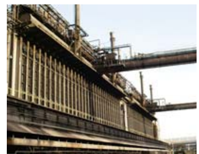
Kakogawa Plant Coke Oven
