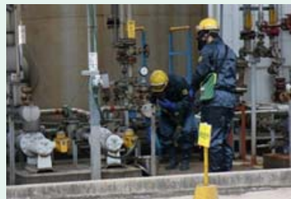
(2) Dealing with a scenario of hazardous item leak at different equipment while the above initial leak is being dealt with
