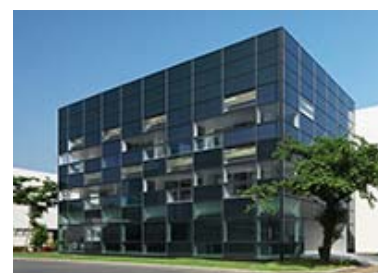
ZEB with film-type OPV units installed on the external walls, Taisei Corporation (Verification test now under way)
