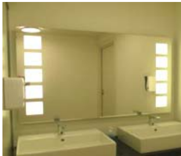
Bathroom vanity washstands
