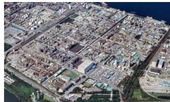
Goi Plant, JPP
