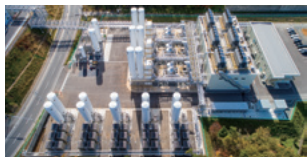
Air separation units (ASUs) that supply highly pure nitrogen in the semiconductor industry
