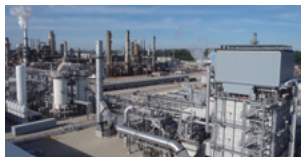
HyCO* plant for hydrogen supply
