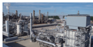
HyCO* plant for hydrogen supply
