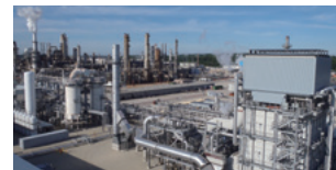
HyCO* plant for hydrogen supply
