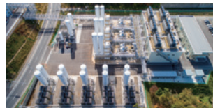
Air separation units (ASUs) that supply highly pure nitrogen in the semiconductor industry
