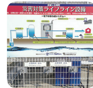
Emergency taps used during the Kumamoto Earthquake and a sign about disaster lifeline facilities (Musashigaoka Hospital)
