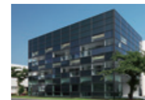
OPV installation example at the ZEB Demonstration Facility (Taisei Corporation)
