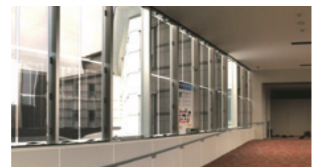
OPV installation example at the Sendai International Center
